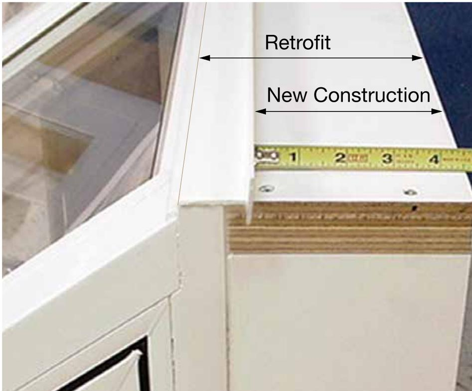
**New Construction:** The flange is installed against the exterior face of the wall (either sheathing or insulation board).
